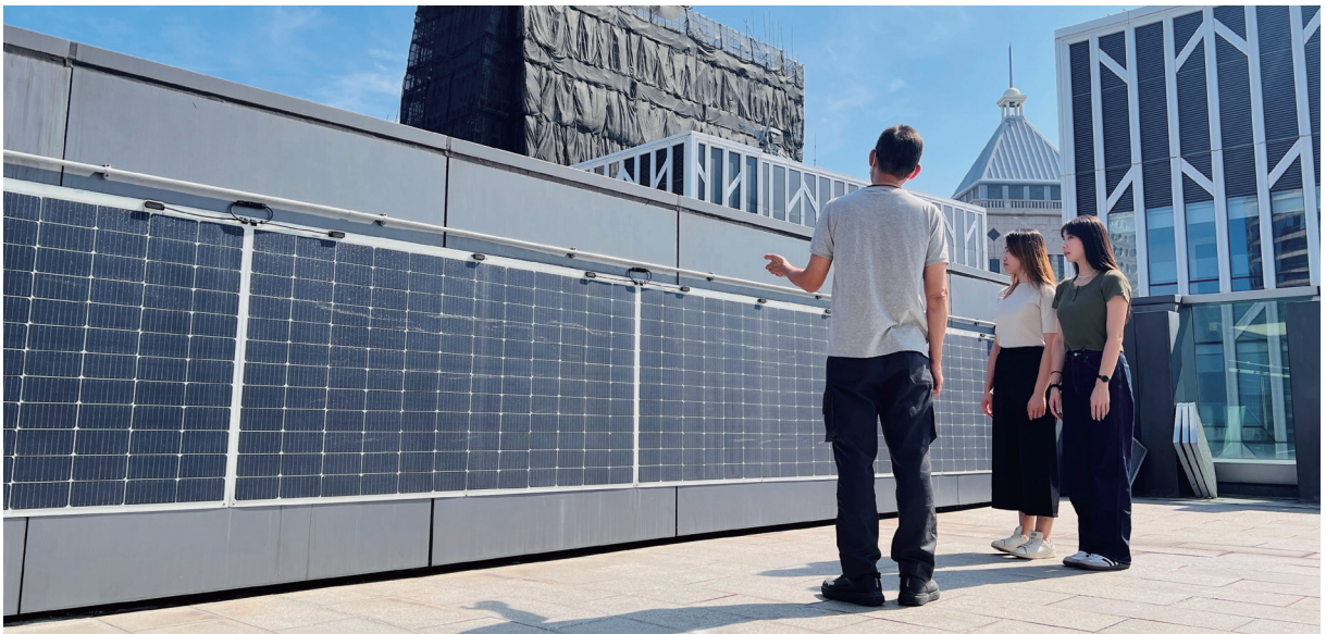
Solar panels were installed at BEA premises to promote renewable energy generation.
